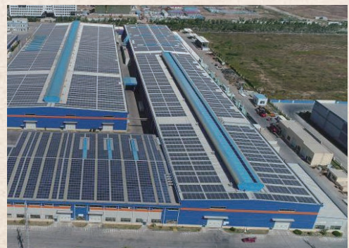
Qingdao Refrigerated Container Base PV Station
